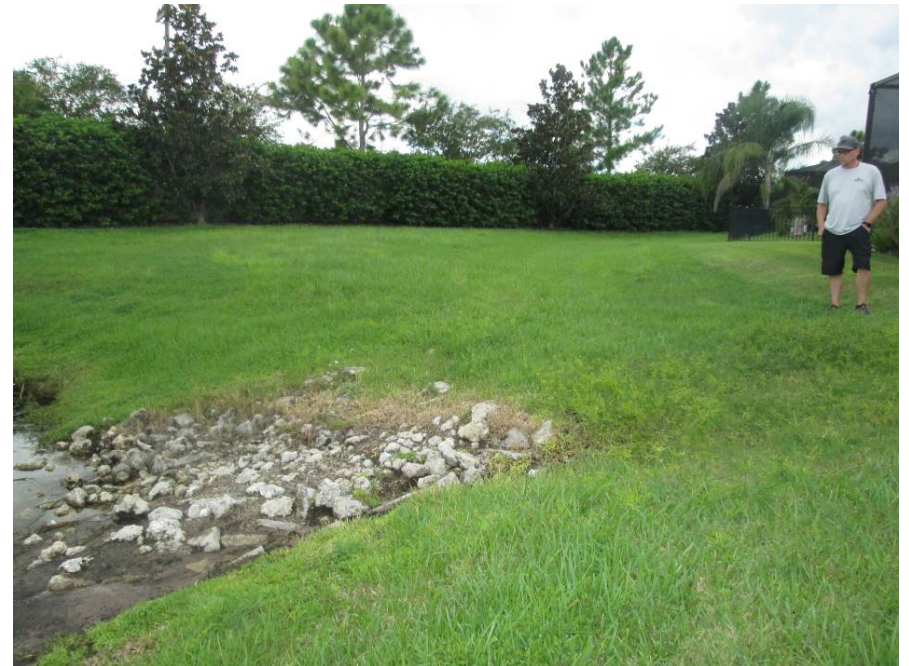
Pond 3 - Southwest corner of pond viewing swale on southwest side
